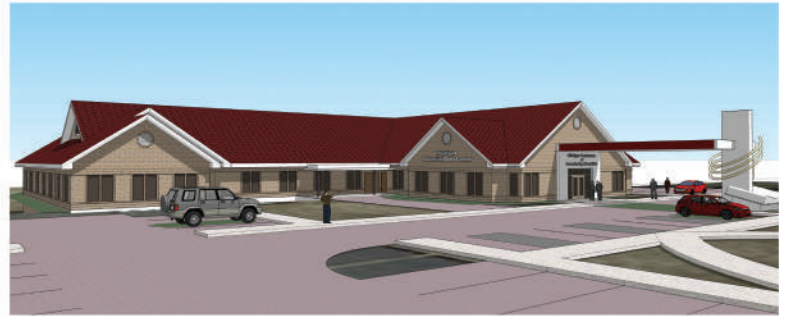
Conference Office view from the northwest
